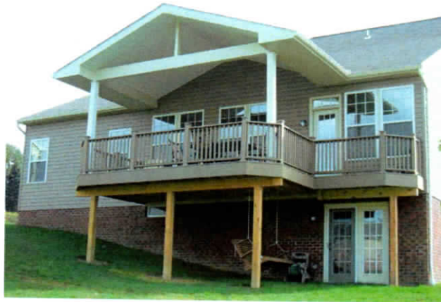
Commonly Referred to as a Gable Style Roof
